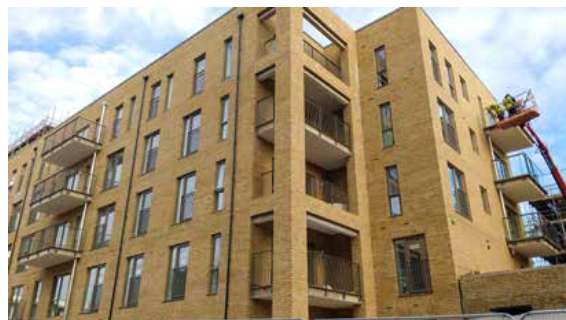
One of the blocks under construction which include the CLT homes at St Clements (Credit: London CLT)
