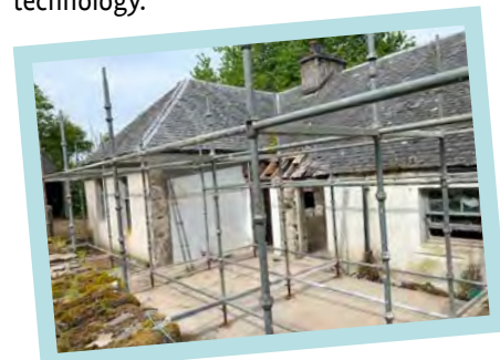
Renovation works on Mull
