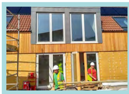
Works underway at Co-housing Bristol
