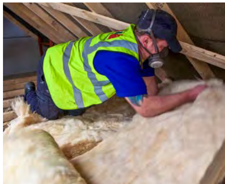
Sustainable loft insulation being installed. Credit: Andrew Aitchison/Alamy Stock Photo
