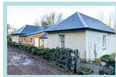
Newly retrofitted homes on Ulva
